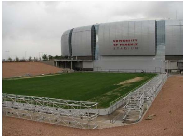
**The new BIRDS NEST** The Arizona Cardinals' \$455 million state-of-the-art stadium is being hailed as one of the top 10 sporting structures in the world. In addition to a retractable roof, it contains the first completely retractable field in the United States.
