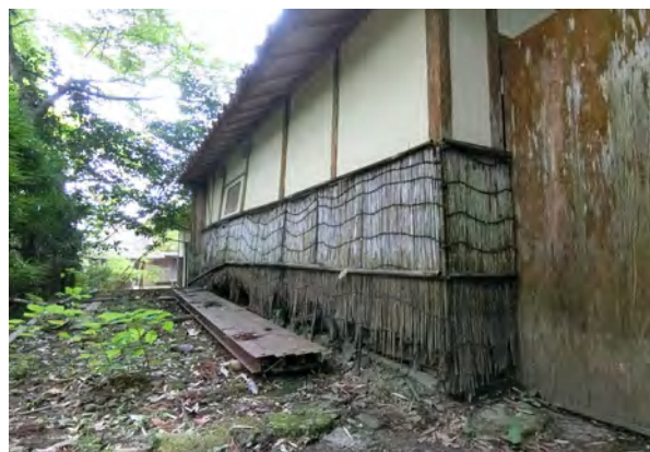
図3-1-30 物置の腐朽
